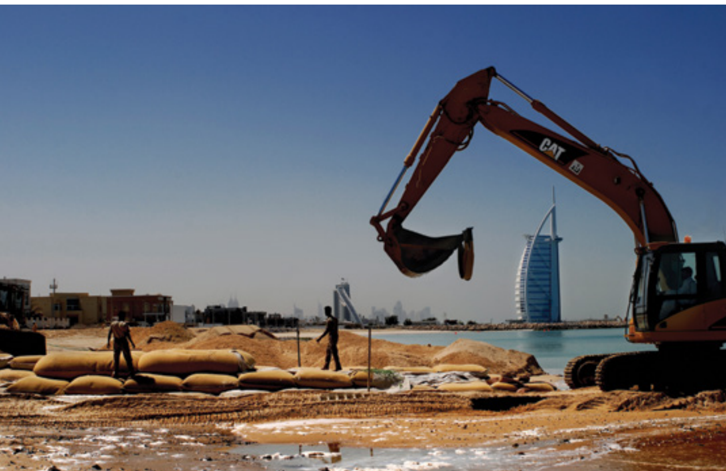
United Arab Emirates (UAE), Dubai. Migrant labourers working on extending the Dubai beach, close to the Burj Al Arab Hotel (right). The employers keep their employees' passports when they arrive and pay their workers around US$167 a month.
